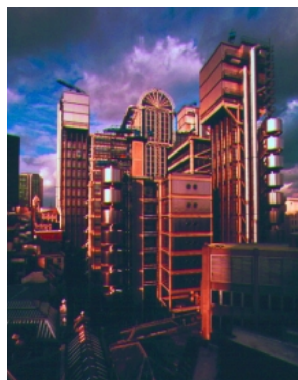
(below) Lloyds of London Building
